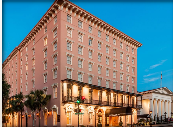
THE MILLS HOUSE HOTEL CHARLESTON
